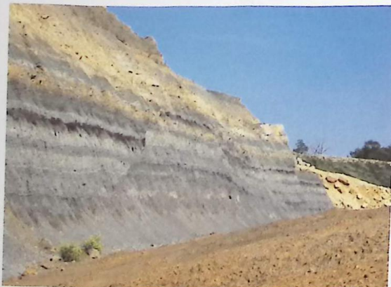
Faulting in the Blisworth Clay (photograph by Fred Owen.)
