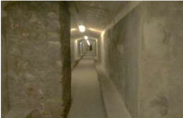
Figure 19: Part of the 4.5km network of tunnels of the Spanish Civil War air-raid shelters which run 9m below the length of the main street in Almeria. They protected about 37,000 people from German and Italian bombing raids. Photo: H.E.Clark
