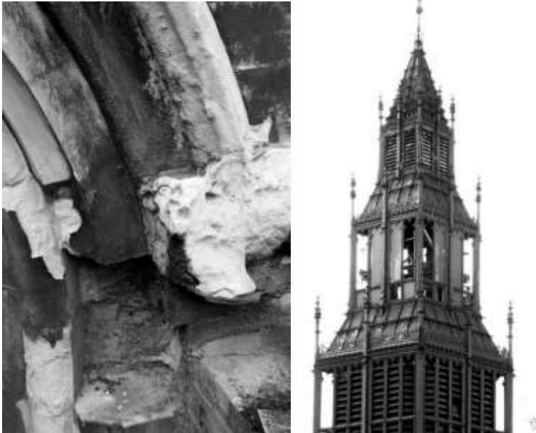
Figure 23: Window surround (left) and cast iron tower (reproduced with permission)
