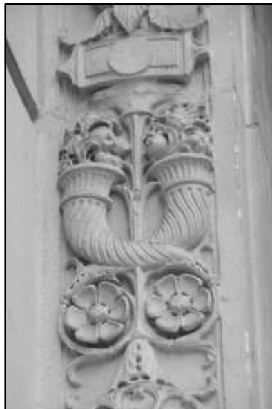
Figure 13: Carving in Portland Stone, Manchester City Centre
