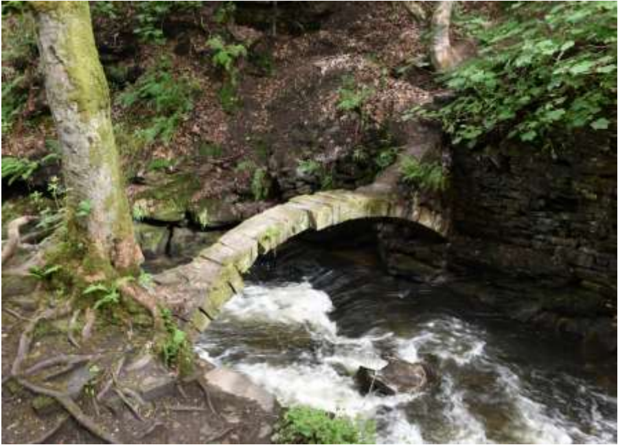
Figure 13: Arch over the Thrutch. Two arches once supported a building (see 10c).
