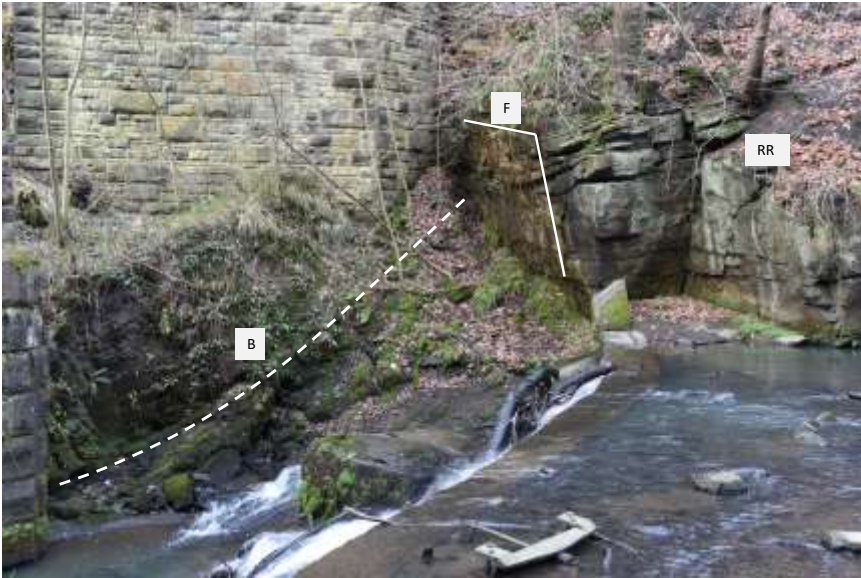
Figure 14: Fault near the abutment of the railway bridge. RR = Rough Rock; F = location of fault plane; B = line following planes of bedding in the shales.
