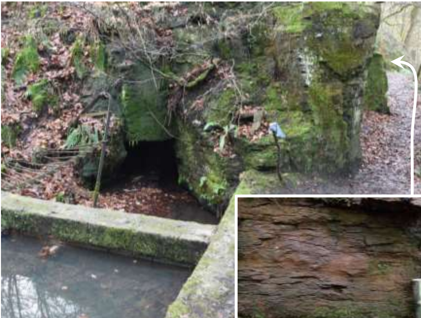
Figure 15: Water flowing from the leat on the left into the tunnel on the right. Inset bottom right: shales – see Location 12
