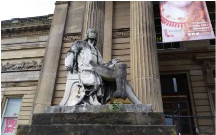
Liverpool: weathering or erosion? https://coord.info/GC744T7
