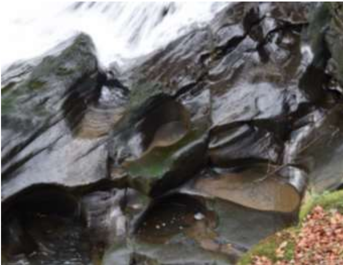
Figure 10: Potholes below the weir (Figure 9)
