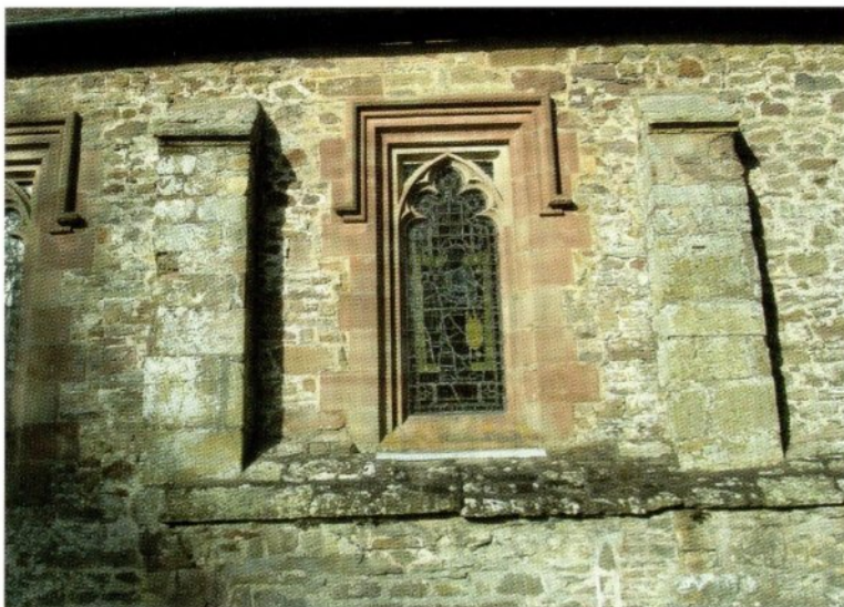
Figure 4 Part of the south wall of Brampton Bryan Parish Church. Finely dressed red sandstones are used for the window. The remainder of the wall is built from the purple Longmyndian sandstones.
