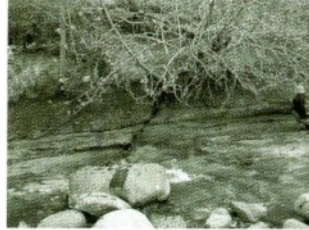
Location 3 unconformity and faulting
